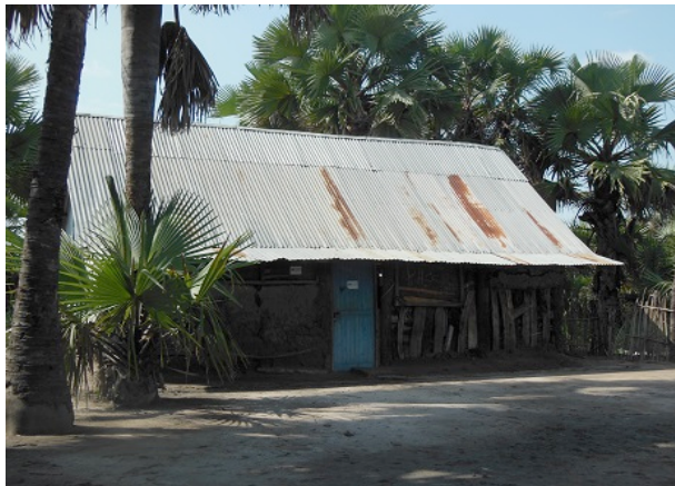
PHCU and compound
