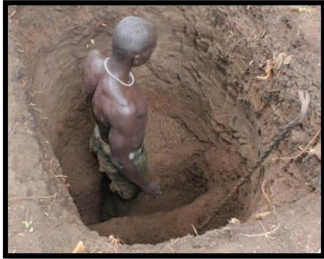
Community members dug a pit latrine for the new school in Pochalla
