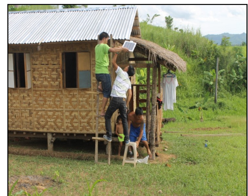
Technicians installing the small solar dish on the roof of a house
